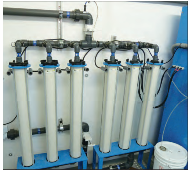
The ElectroPulse system from OilTrap Environmental (Tumwater, Washington) is wired to a central control panel (left). It adjusts the pH of the wastewater before sending it through a series of 4"-diameter (102mm) tubes fitted with electrically charged plates (right) that change the polarity of any suspended solids, causing them to cluster and float, and rendering any metals inert through oxidization.
