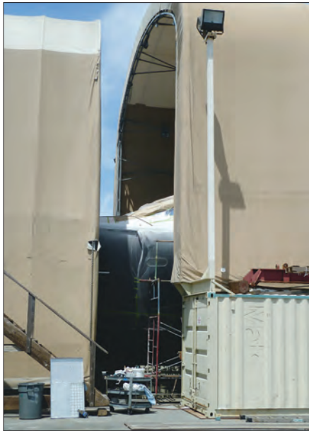
A temporary fabric-covered structure welded to a surplus Travelift (seen at left) can be driven anywhere in the yard to shelter a project. Here, it covers the bow section of a Sunseeker that can't be fully enclosed by the less-mobile fabric-covered structure that's anchored to shipping containers at yard level.
