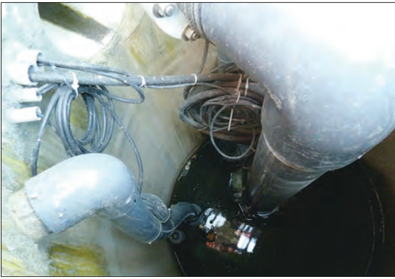
Left —Storm water from the entire 68,000-sq-ft (6,317m 2 ) Sausalito yard ends up in this 1,000-gallon (3,785-l) settling tank, affectionately referred to as “the wishing well.” From there, three pumps of varying capacities pump it up to a rooftop Aquip system from StormwaterRX (Portland, Oregon), capable of filtering 110 gal (416.4 l) per minute. Right —Samples of treated and untreated water and the five filter media in the Aquip filter tank. Treated stormwater can be discharged directly into the bay.
